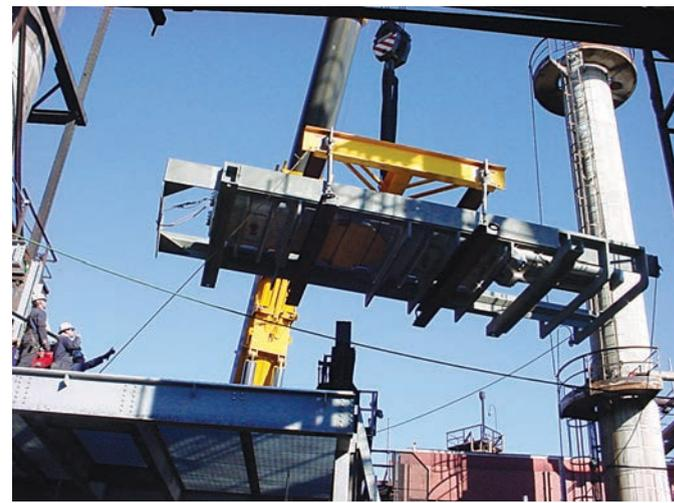
A Delta valve is lifted into a structure using the Delta Glide System, while AltairStrickland personnel oversee the work.
