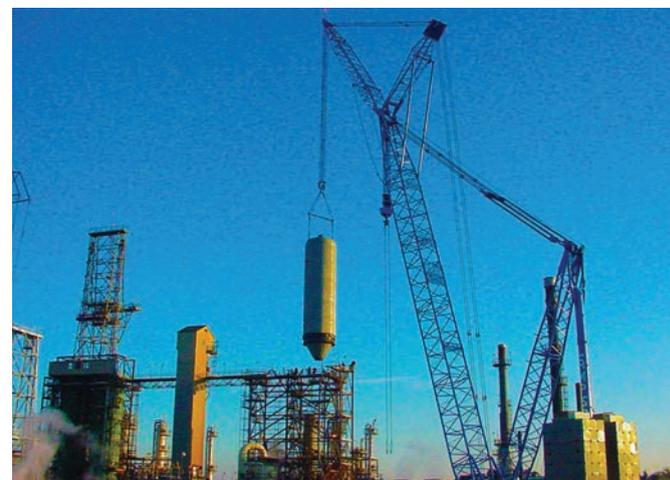
A crane lifts a new coke drum into a structure during one of AltairStrickland’s turnarounds.
